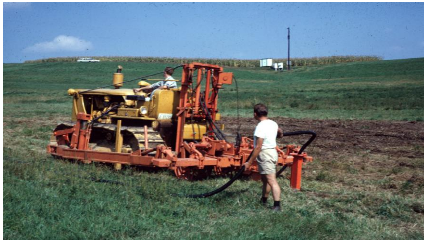
Fig. 1. Small-Diameter Corrugated-Wall Plastic Drain Tubing being Plowed-In behind a Mole-Plow; 1965, Coshocton, OH.
