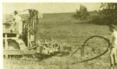
FIG. 3 Corrugated plastic drain tubing being installed with hollow-bladed tool drawn behind a mole plow. This material could be fed from a coil mounted on the equipment
