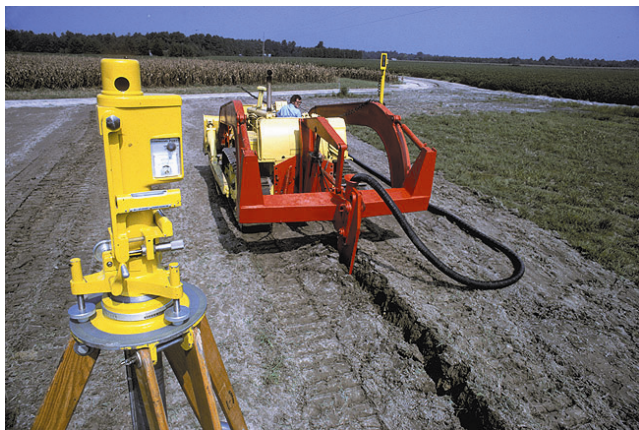
Figure 5. ARS experimental draintube plow with Laserplane automatic grade-control system installing 100 mm drain.
