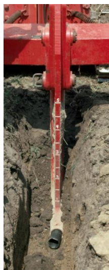
Plow Starter Trench at Main
