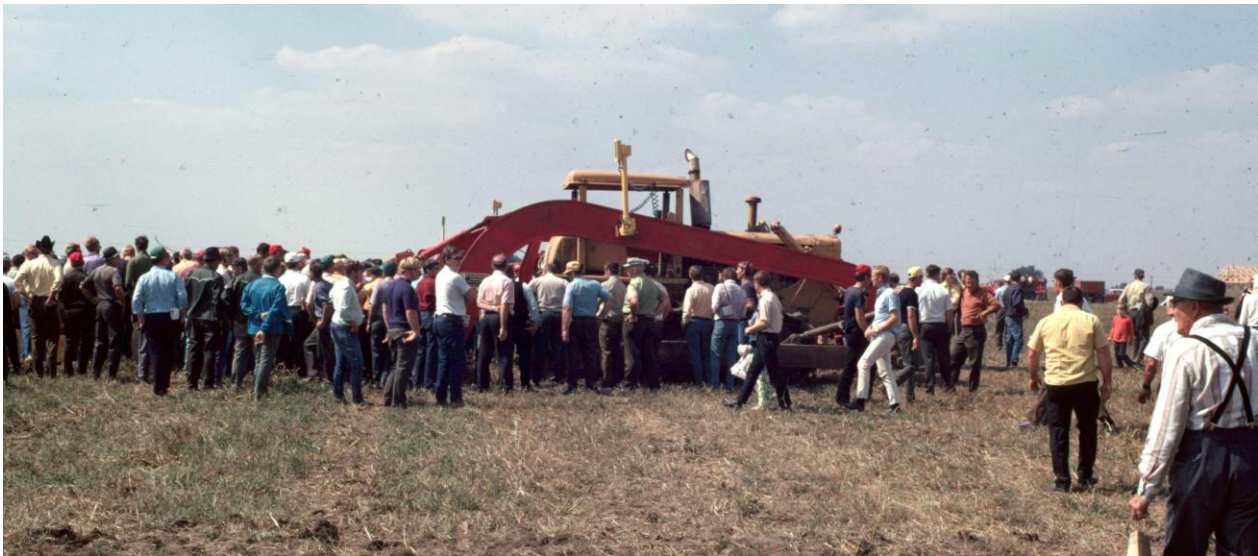
Drainage contractors, farmers, and drainage industry representatives observing the ARS Big Red Plow installing corrugated plastic drain tubing at 1971 OSU Farm Science Review
