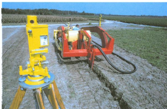
Figure 5. ARS experimental draintube plow with Laserplane automatic grade-control system installing 100 mm drain.
