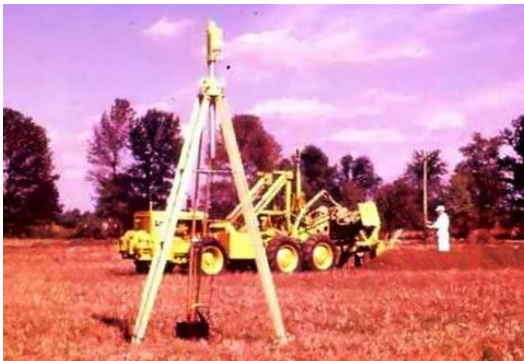
Fig. 24. First public field demo of Laserplane Grade-Control system on a Drainage Trenching Machine at the Ohio State Farm Science Review, Fall of 1968.
