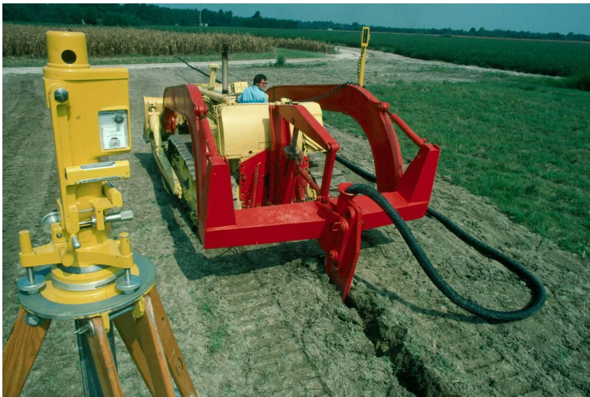
Fig. 25. ARS “Big Red” Draitube Plow with Laserplane Depth & Grade-Control System Mounted on a D-7E CAT Installing 4-in. dia. Corrugated-Wall Plastic Draitube.
