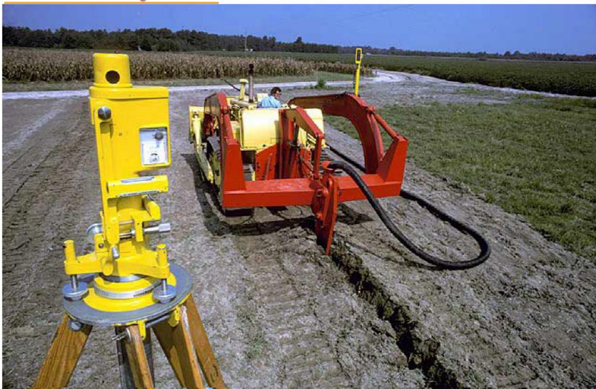
Figure 2. Laser-controlled ARS draitube plow.
