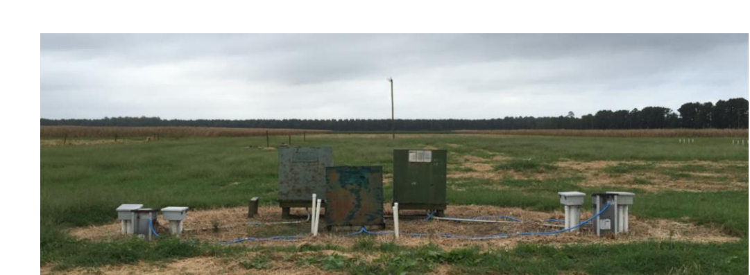
Fig. 3 Flow and water quality measurement equipment
